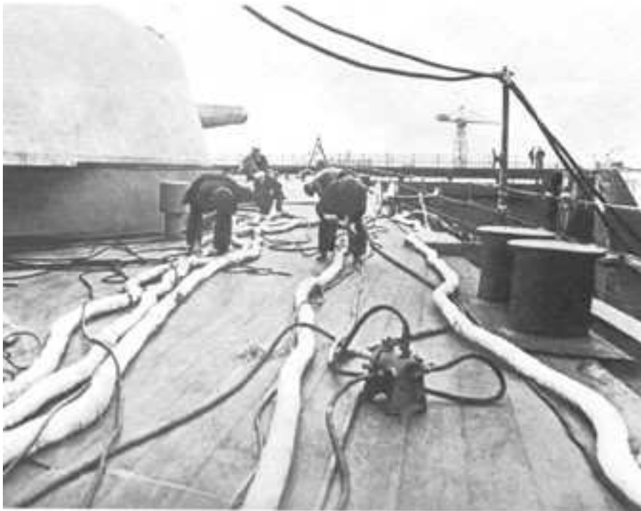
Sailors laying down degaussing coils on the deck of a warship ( contr. by Akronos Publishing )
